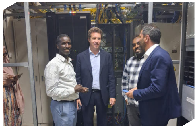
Executive Director, Umberto Tavolato, leads a Med-Or Africa team during a visit to the datacenter at a submarine cable landing station in Djibouti.
